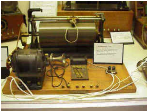
Magnetic wire recording by V. Poulsen (1898),
