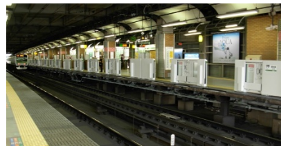
Application to platform door (JR Ebisu station)
