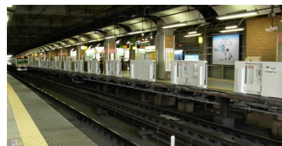
Application to platform door (JR Ebisu station)
