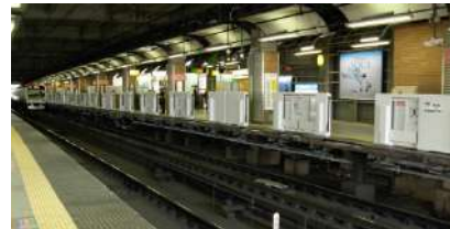
Application to platform door (JR Ebisu station)
